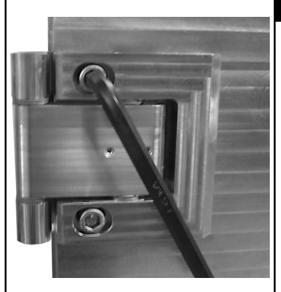
With the door still open and while someone continues to hold the latch side of the door, loosen the upper screw on the top hinge.
