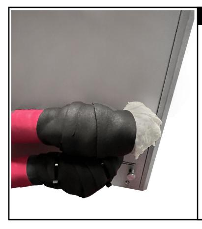
Continue wrapping Armaflex strips over the ceramic insulation.
