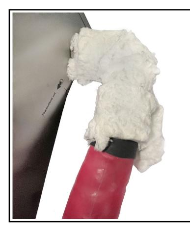
Finish wrapping the insulation so that it completely covers all exposed pipe including over the reduced diameter section of the Swagelok hose.
