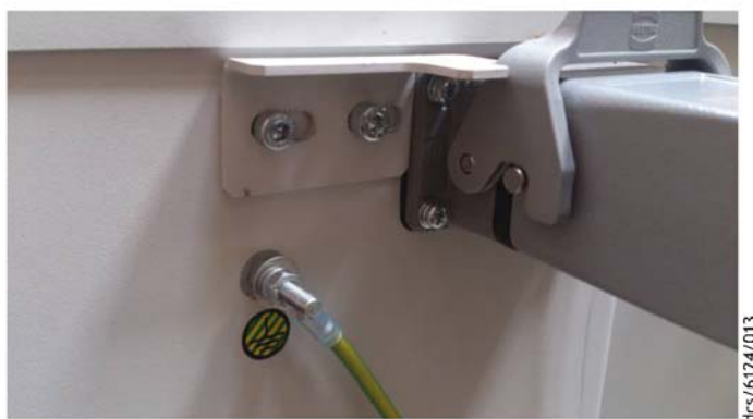
Figure 12 - Protective Earth (PE) connection
