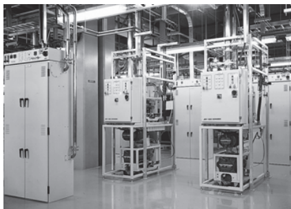
GRC technology has been used to abate the exhaust gas streams on a wide range of semiconductor applications. (Photograph courtesy of TI, Dallas, USA.)
