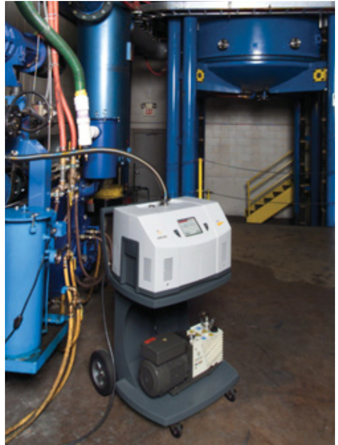
Leak Detection application. Photo courtesy Carbon Composites.
